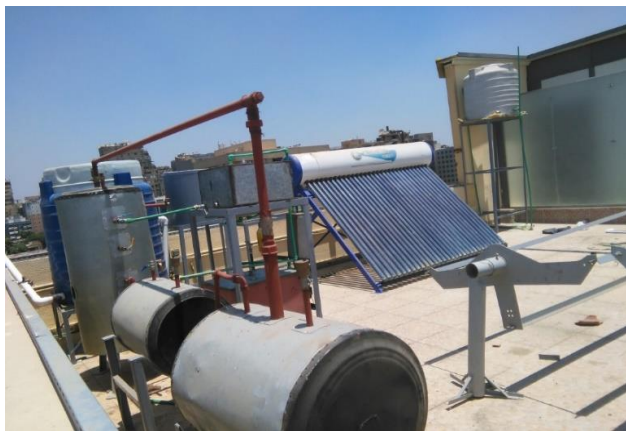
Fig. 1 Solar water desalination system using evacuated tube collector
