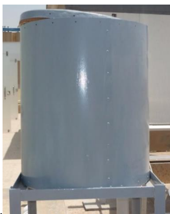
Fig. 5 The supplementary hot oil electric heater storage tank
